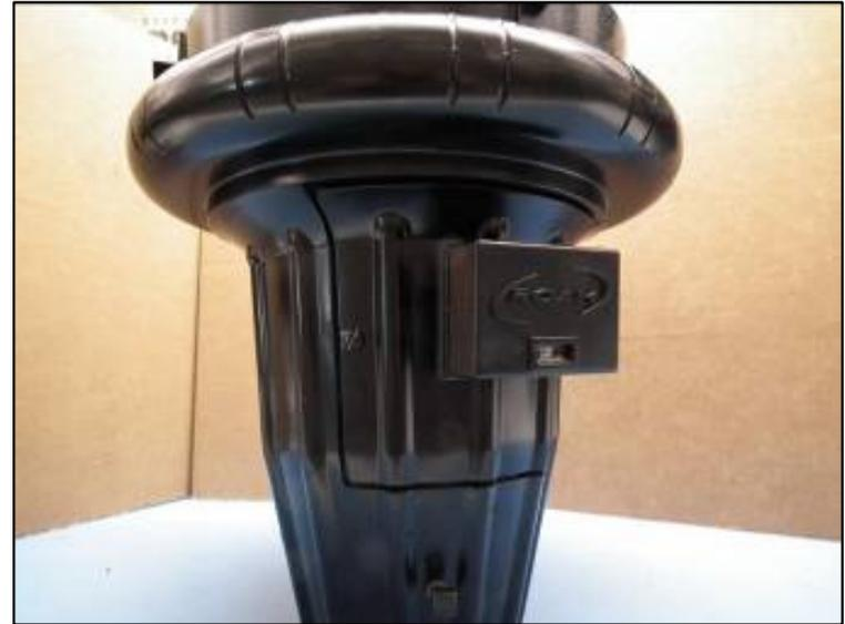
16. Deco Utility photocontrol installation is now complete. Different methods may be employed to electrically test the fixture or proof the wiring at this point. Due to differences in manufacturing processes and fixtures, the remaining steps are included only as an example of possible fixture tests.
