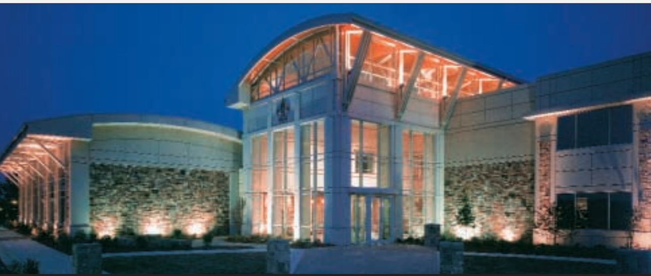
Boy Scouts of America recently opened a new Volunteer Service Center in Atlanta, Georgia. Enhancing this magnificent structure are ALG indoor and outdoor lighting fixtures.
