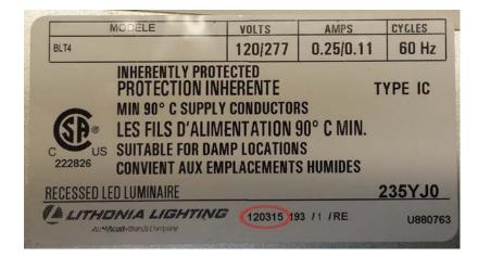
The date code on the fixture's housing's label is in a MM/DD/YY format.
