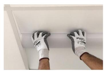
B. Lens will begin to disengage. Work lens loose and remove from fixture. After removal, set aside in a safe area for later use in Step 5A.
